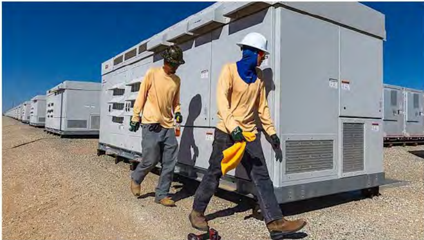
Technicians install equipment at a Solar Power/Battery Energy Storage System in San Bernardino County, 2023. [Photo: Irfan Khan/Los Angeles Times/Getty Images]
